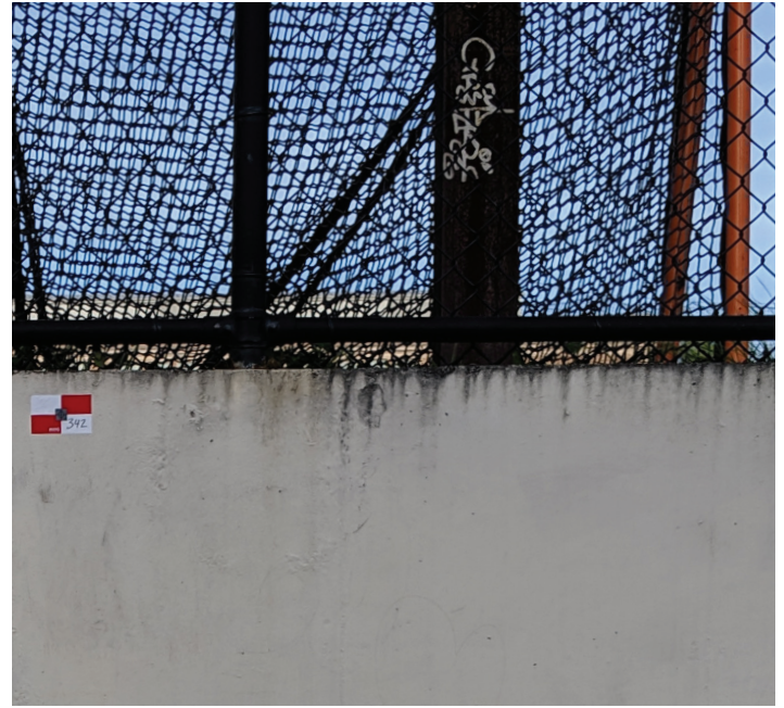
Optical target on a retaining wall.
