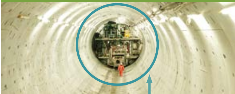
If you look closely, you can see the rings that were placed by this TBM to form the "Lee Tunnel" in London.
